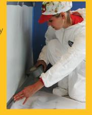
Make a curtain by taping plastic sheeting over the doorway to the work area.
