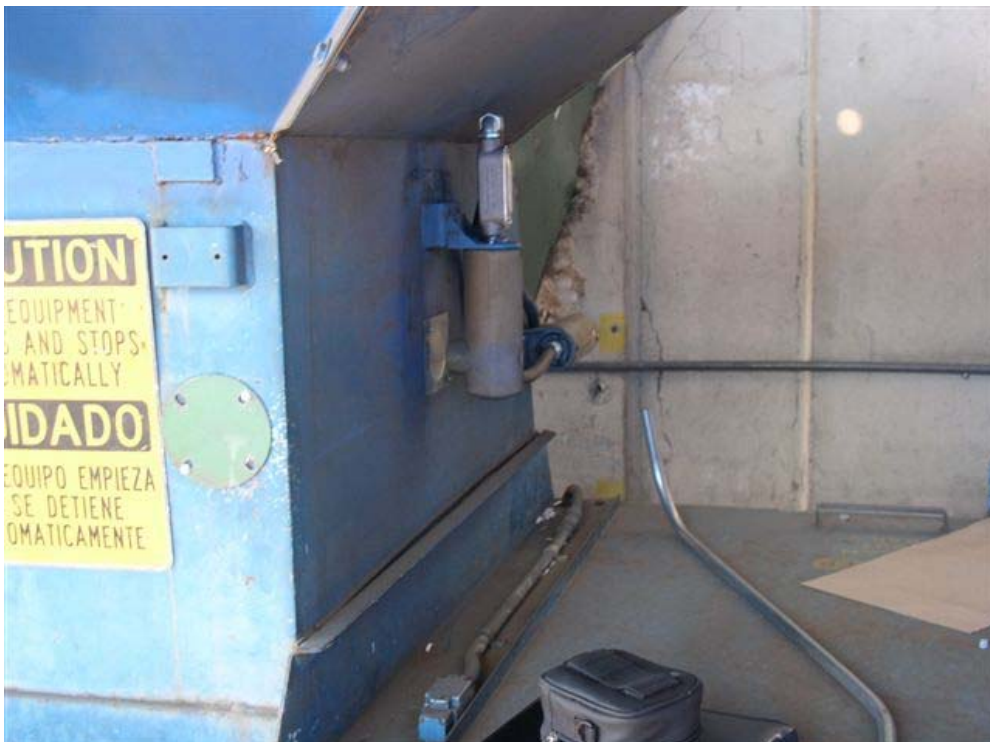
Exhibit 6. The electronic sensor on the feed hopper.
