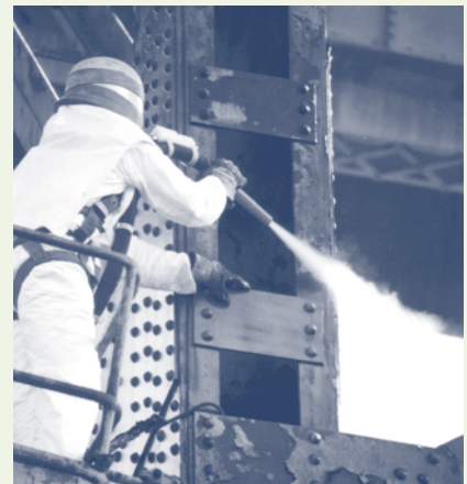
Industrial painter using a wet blasting removal method
