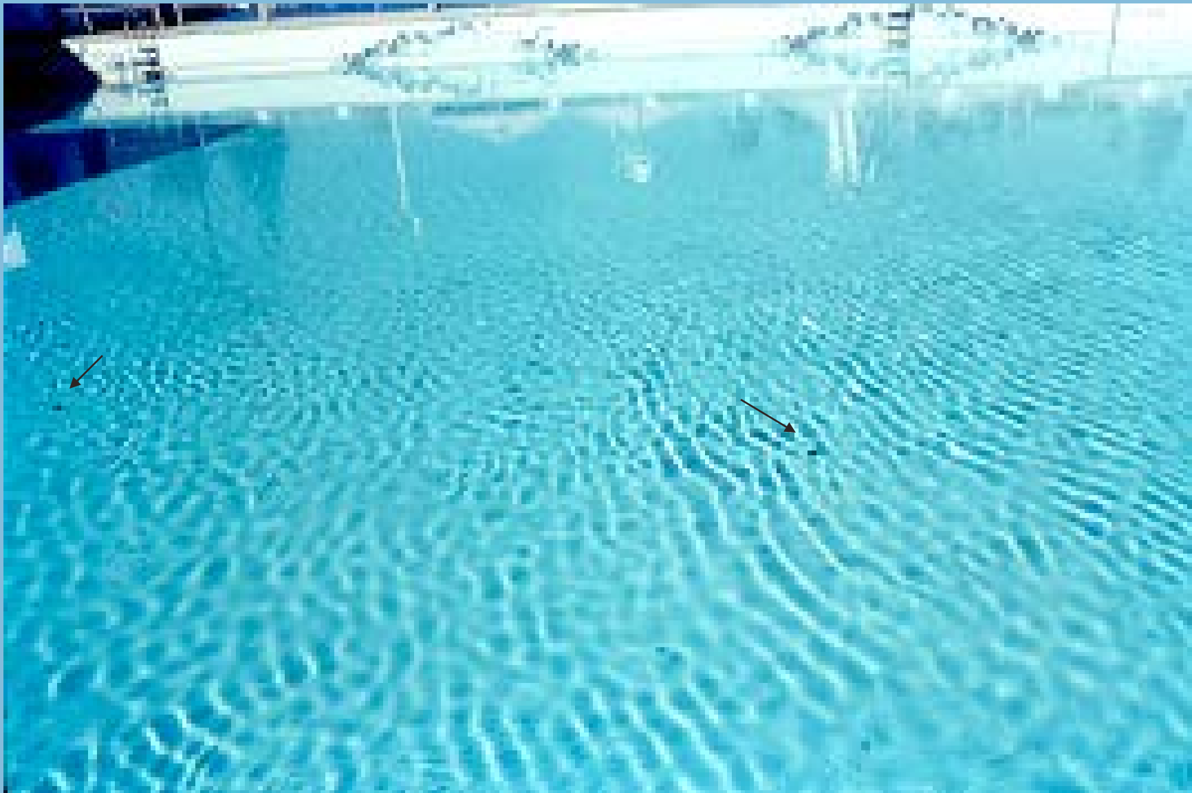
Oasis Water Park- missing main drain covers
