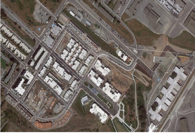
Figure 2: Aerial view of Parcel A1 with buildings surveyed
